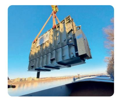
Transformers can be transported completely filled with or without oil in the main tank, depending on the size.
